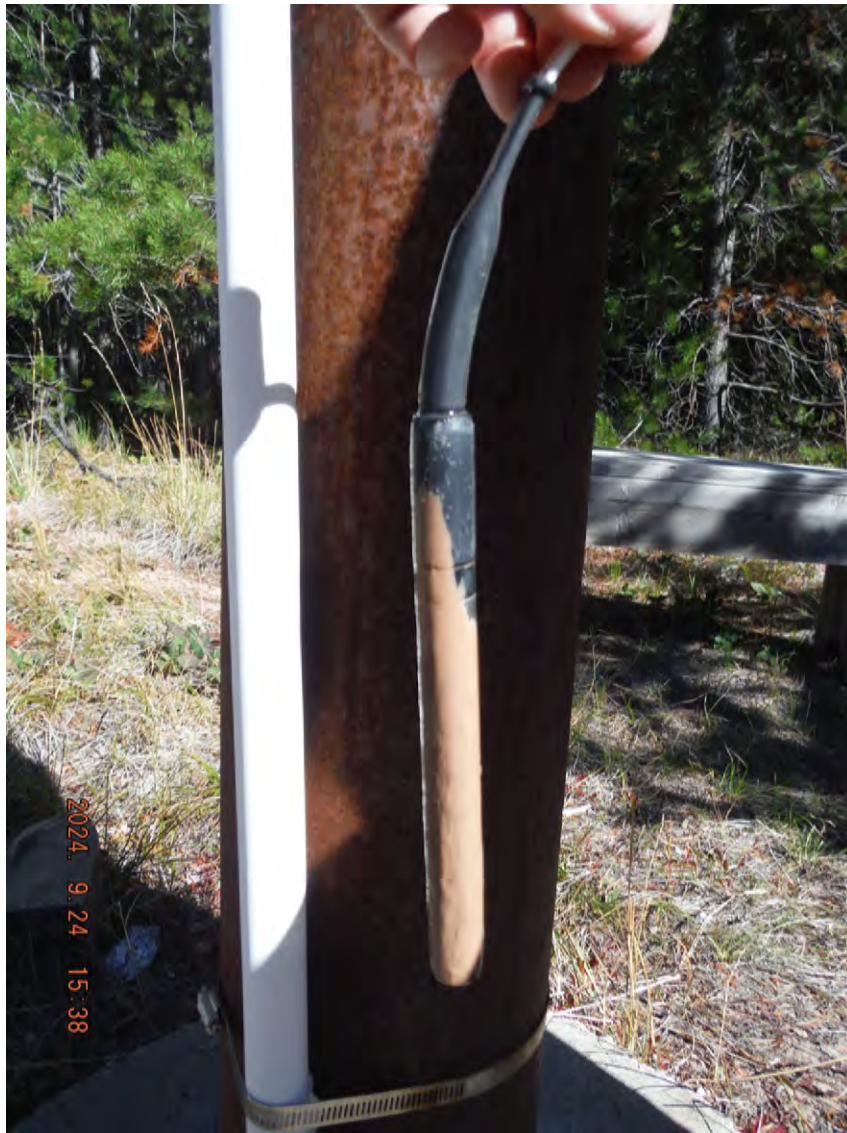
Sediment Accumulation in Monitoring Well S35-MW-03, September 2024
