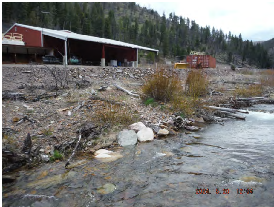
No Flow in Water Treatment Plant Outfall Channel Entering the Blackfoot River, May 2024
